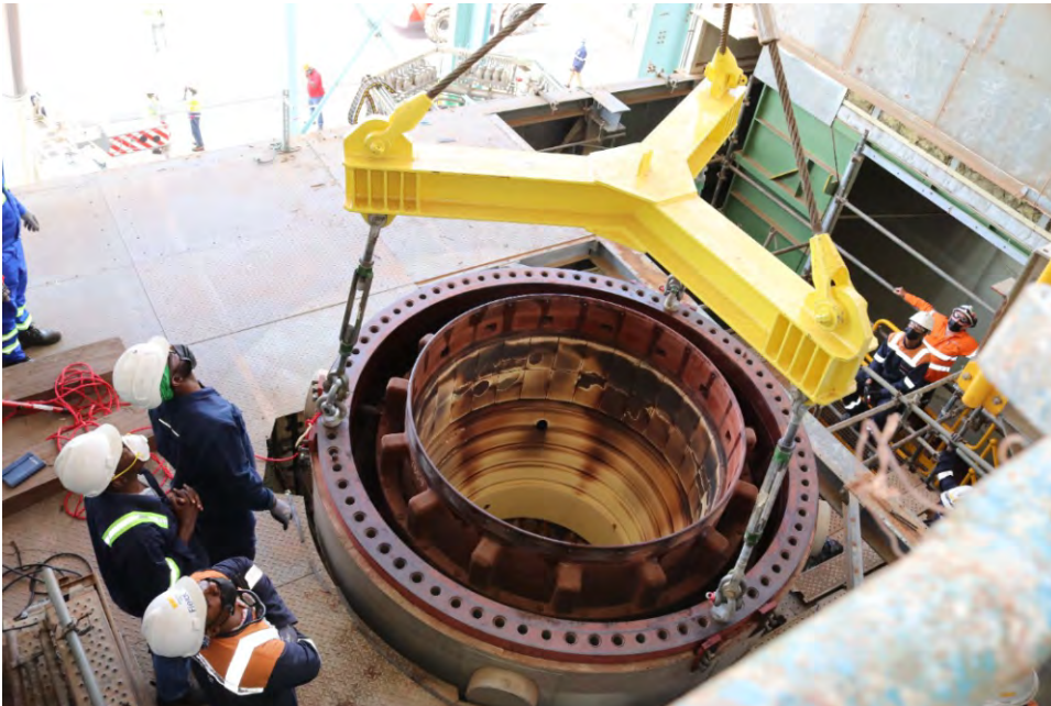
Removal of the Combustion Pot
